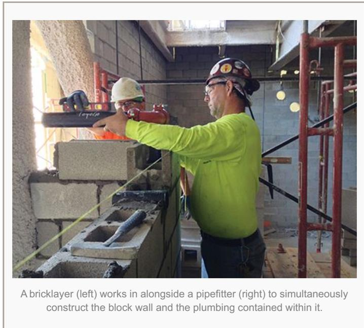
A bricklayer (left) works in alongside a pipefitter (right) to simultaneously construct the block wall and the plumbing contained within it.
