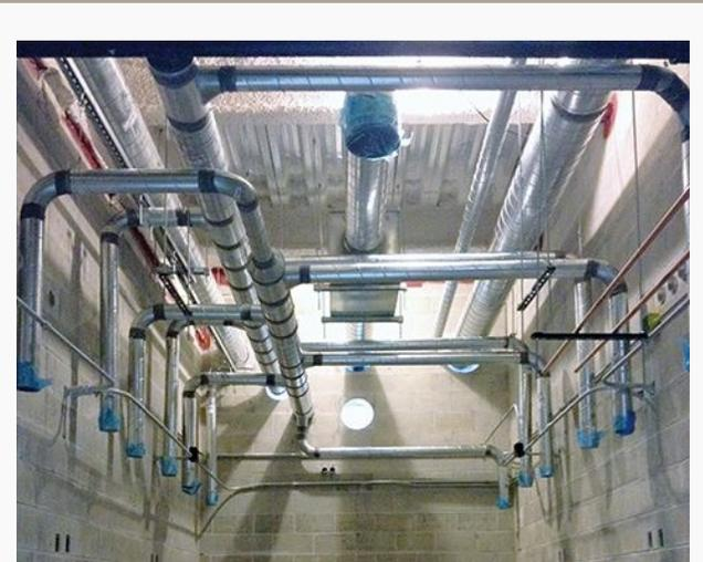
Upon completion of the masonry work, the MEP trades were able to easily install their pipes and ducts without cutting through the masonry due to the well-coordinated sleeve penetrations.
