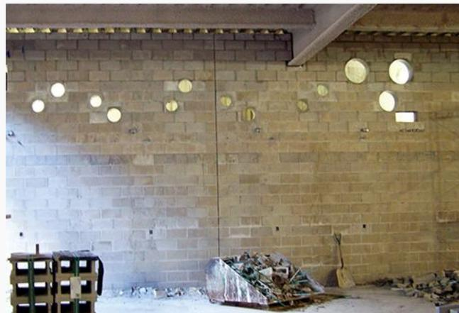
As the concrete masonry wall was constructed, the bricklayers installed 468 sleeves for fire protection, 231 sleeves for plumbing, 343 sleeves for water, and 10 miscellaneous sleeves. There was a total of 1537 sleeves.
