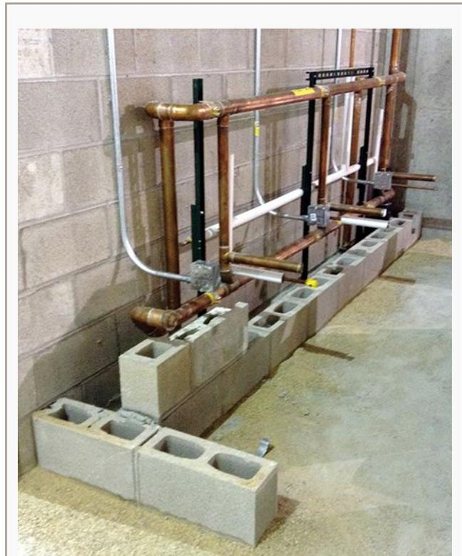
The BIM model made it possible to prefabricate the toilet room plumbing assemblies on steel strut racks to conserve space onsite. The plumbing racks were integrated into the block walls per the coordination model.
