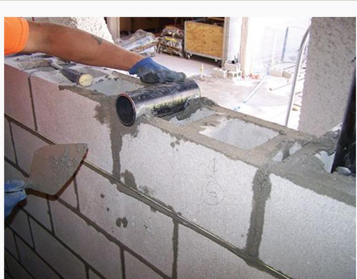
For this project, the bricklayers worked alongside the mechanical, electrical, and plumbing (MEP) trades to install pipe sleeves through the masonry walls as they were constructed, per the BIM model.
