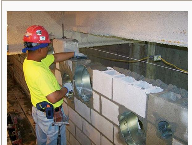
In the photo above, a bricklayer installs mechanical duct sleeves at precise locations per the BIM model, as he constructs the masonry.
