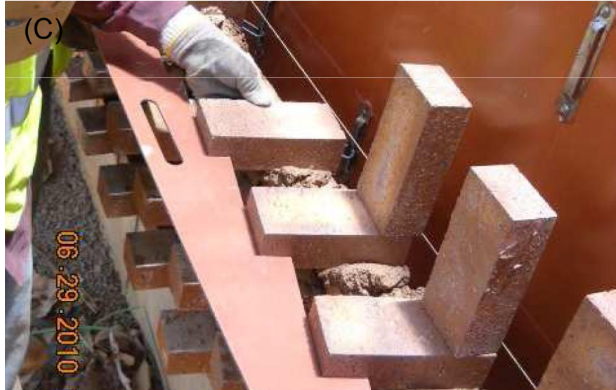
Figure 4: (A) Southern Polytechnic State University, Design Studio II, by Cooper Carry Architects, (B) conceptual strategy of brick coursework, (C) templating of rotating brick during construction (image credit: Cooper Carry Architects).
